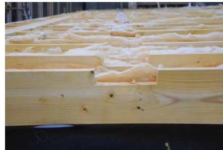
The Joists are notched for the pipework to be laid (above)
