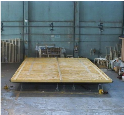
Joists are laid then the base is insulated (above)
